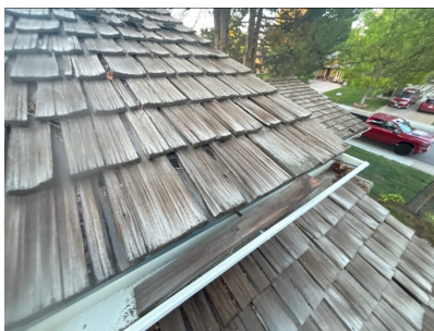
PHOTO 10 / GUTTER AND SHAKE EDGE
