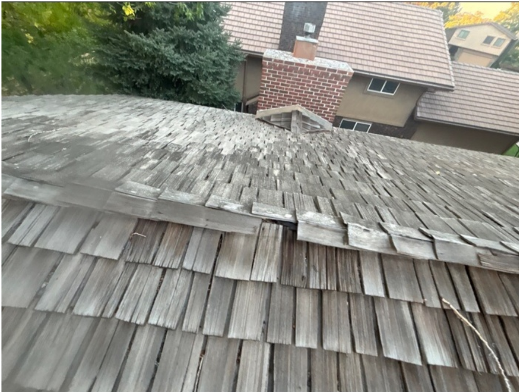
PHOTO 11 / OPEN CAP JOINT
