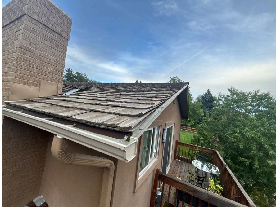
PHOTO 06 / UPPER GUTTER CONNECTION
